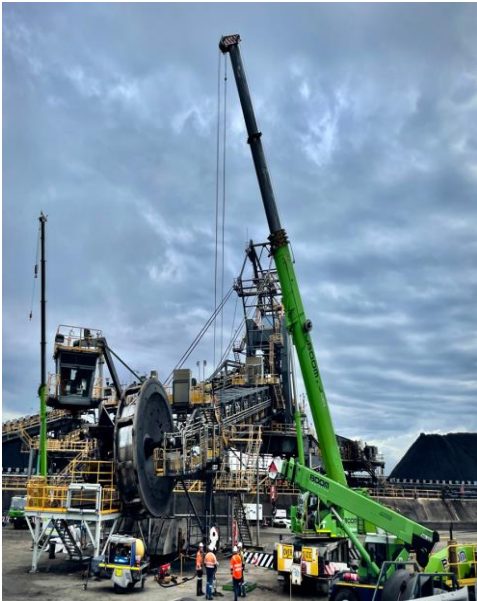
BMA Hay Point Shutdown works 130t & 80t All Terrains + 25t Franna
