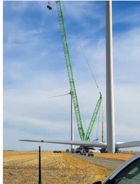
Murra Warra Wind Farm Western Victoria VIC Turbine construction project 250t & 500t All Terrains
